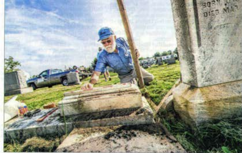
Ted Kusters of Abba Monument Co. in Newark uses a level to check the base of a grave marker he is repairing at Riverview Cemetery in Wilmington. ROBERT CRAIG/THE NEWS JOURNAL
